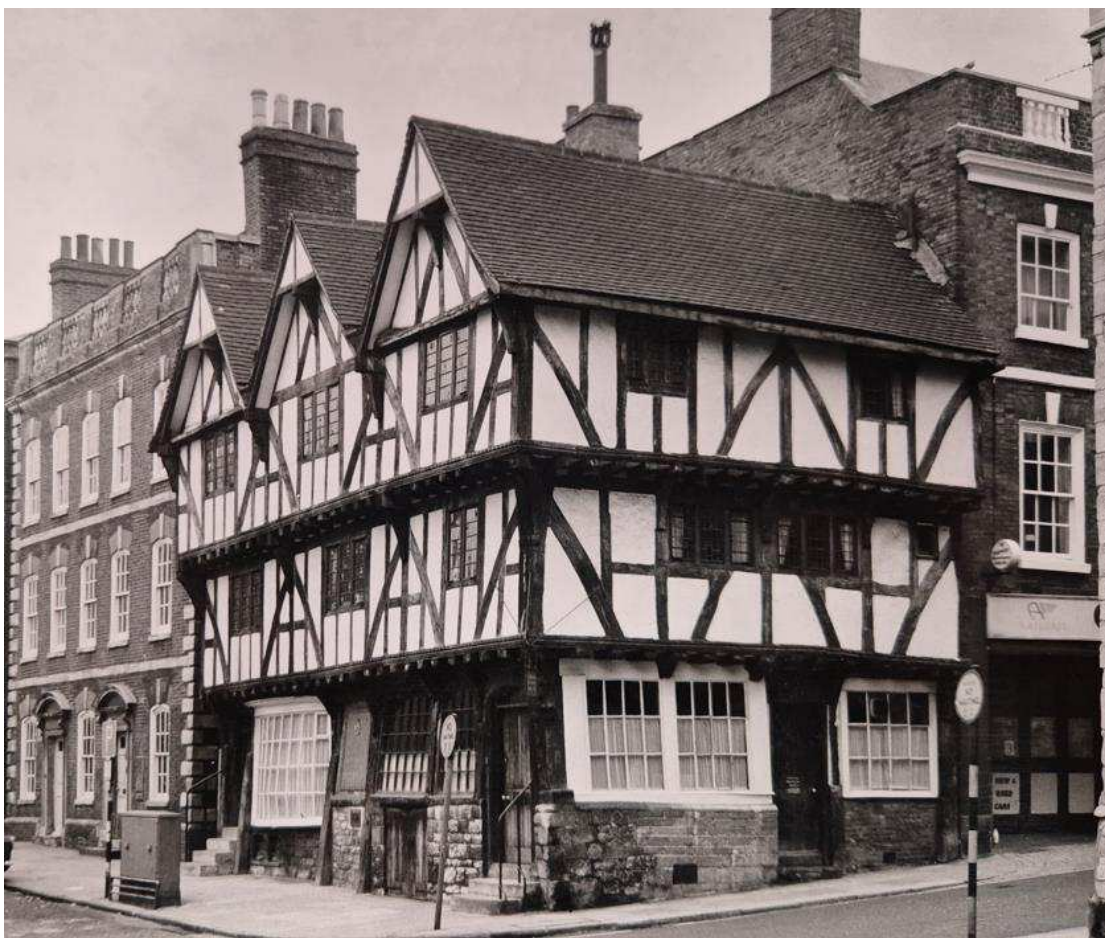
Figure 35 1967 image looking northwest to the corner of the building. 73
