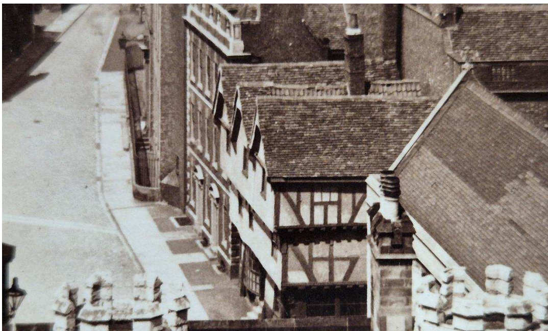
Figure 15 Extract from a c.1900 images taken from the cathedral showing plain clay tile and pantile roofing on the building. 37
