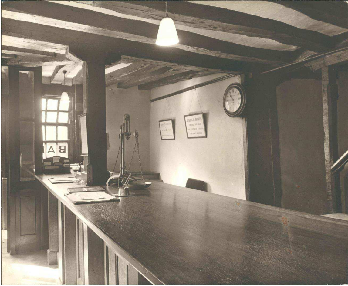
Figure 25 1930s interior of the banking chamber looking southwest. 55
