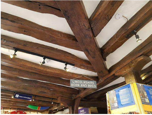
Figure 51 Looking northwest (L) and southeast (R) to the ceiling framing of the east side of the ground floor including diagonal dragon beam.
