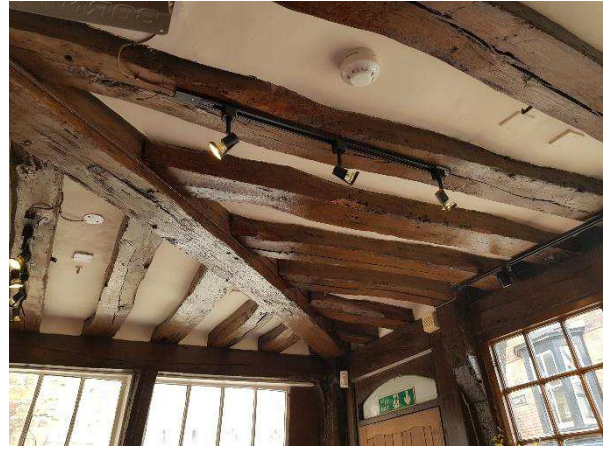
Figure 51 Looking northwest (L) and southeast (R) to the ceiling framing of the east side of the ground floor including diagonal dragon beam.
