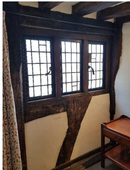
Figure 65 Detail of the small 20 th century window to a possible former toilet in this corner(L) and 20 th century casement windows (replaced a Yorkshire sliding sash window) (R) in the northeast corner room east wall.
