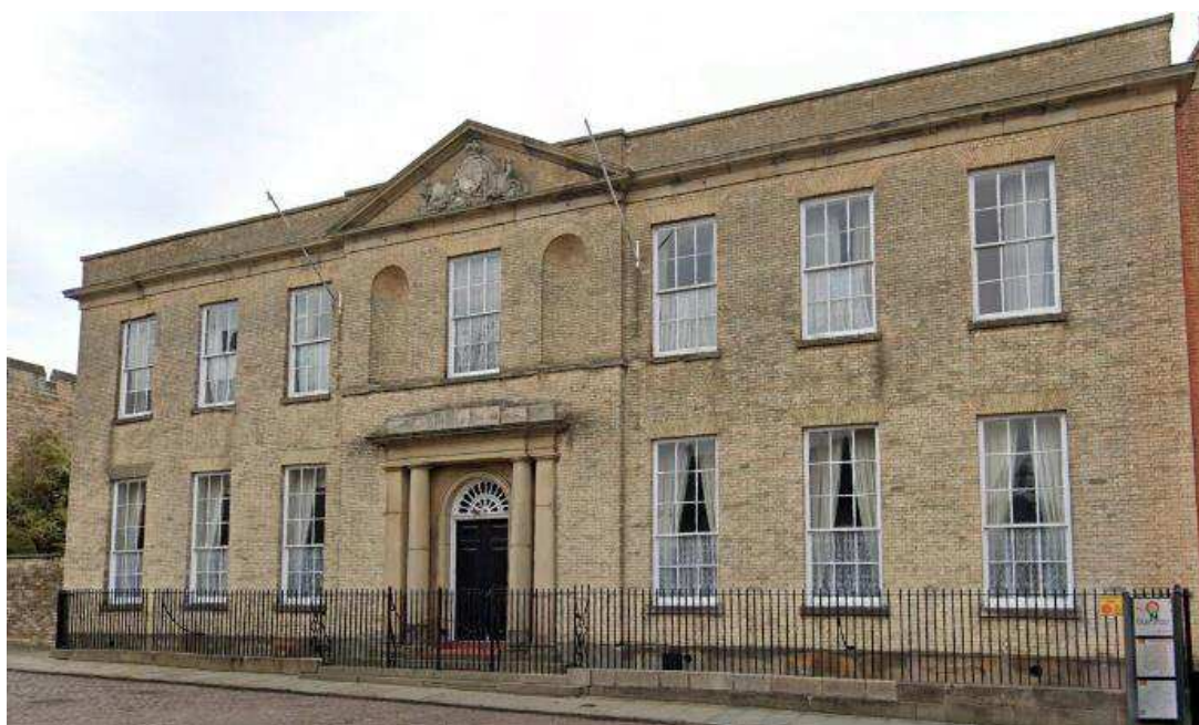
Figure 89 South elevation of the Judges Lodgings on Castle Hill. 92
