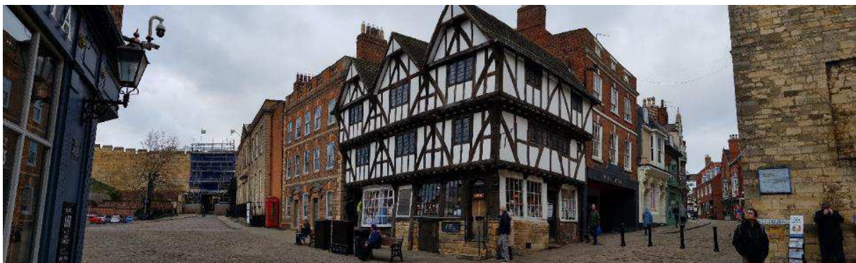
Figure 1 Panoramic view looking in a north-westerly direction showing Leigh-Pemberton House forming the northwest corner of the junction between Castle Hill (to the left) and Bailgate (to the right).
