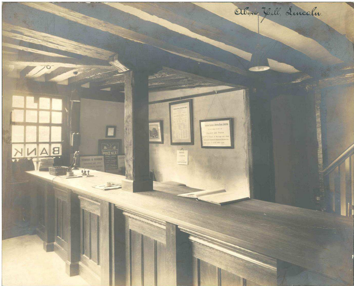
Figure 17 1912-1923 interior photo looking southwest in the ground floor banking chamber of the east tenement. 45
