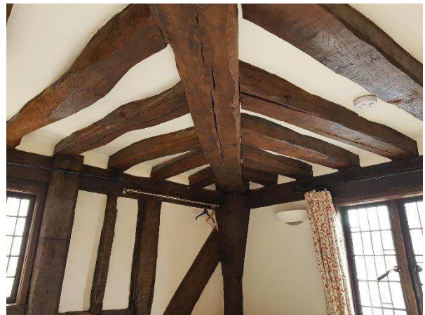
Figure 62 Looking east (L) and southeast (R) in the southeast corner room including corner dragon beam.
