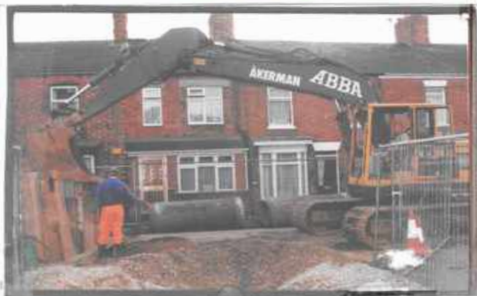
Archive picture of Sewer work on West Parade
