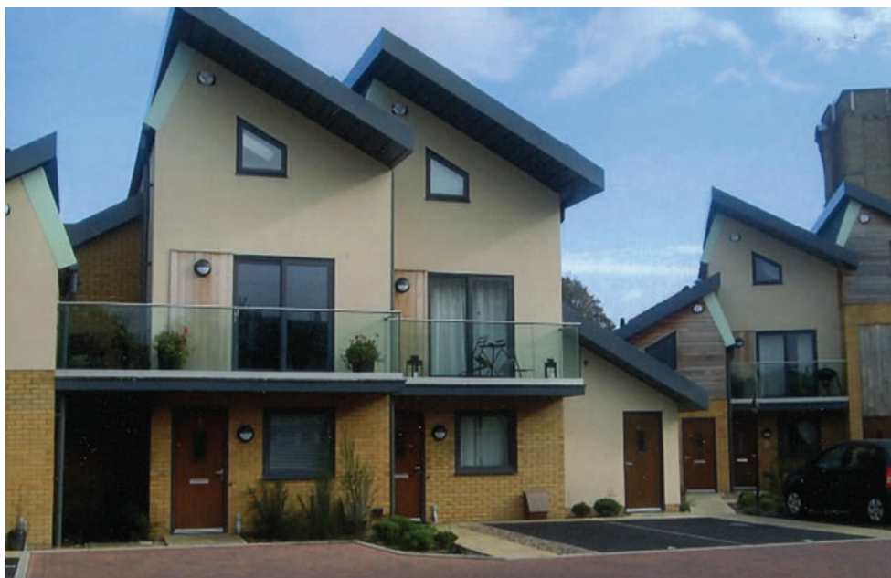
Cuthberts Yard, Burton Road (Oasis Design & Architecture)
